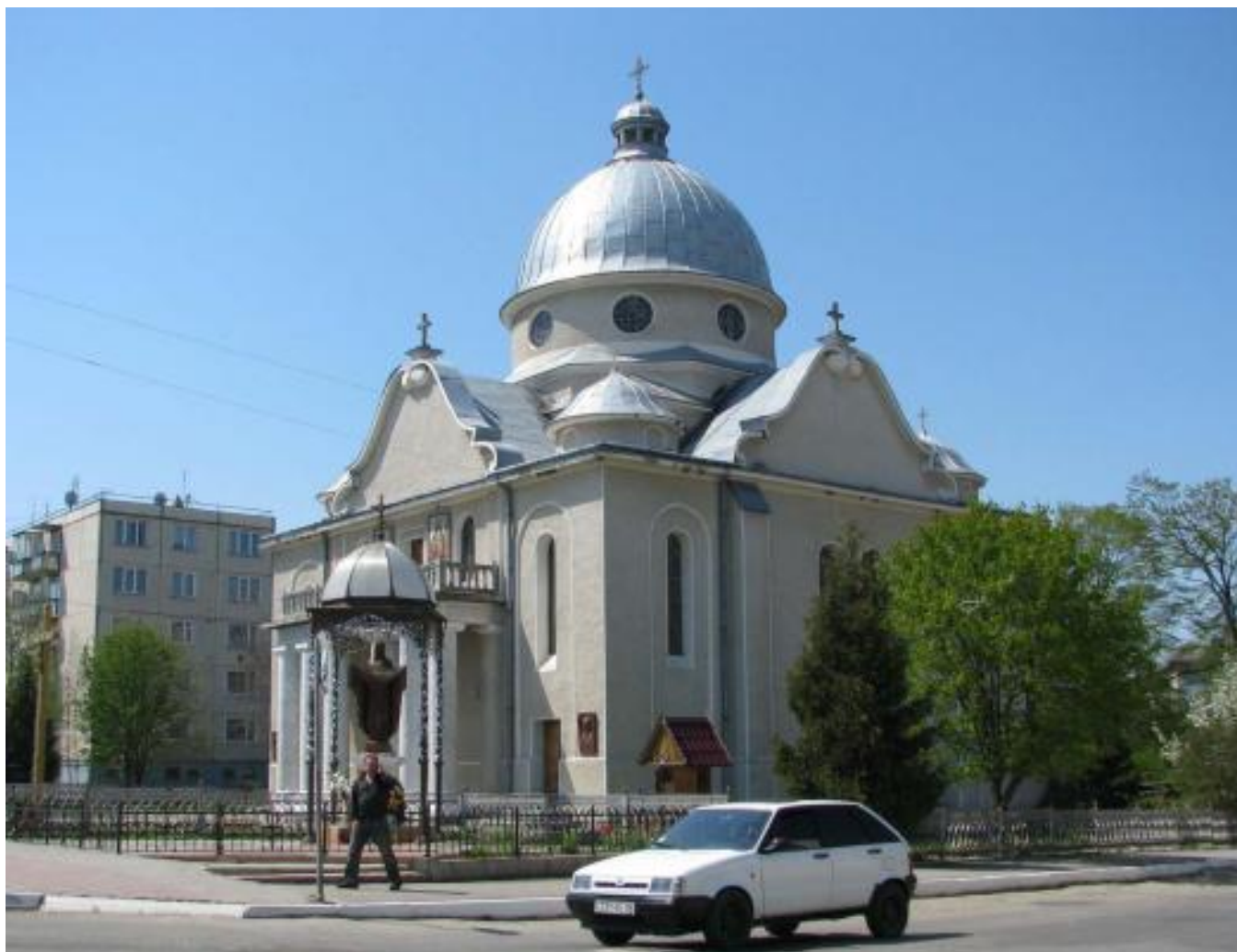
Bohorodczany, general view
